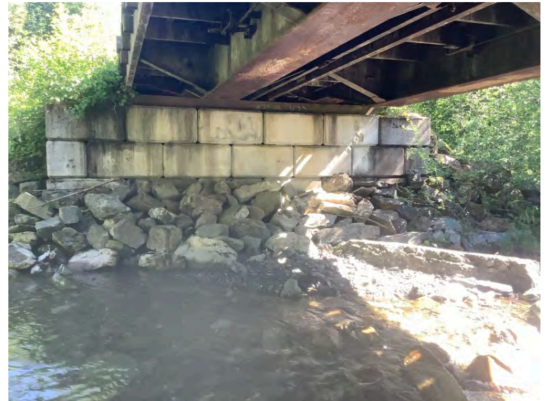
Left Bank Abutment when facing downstream
