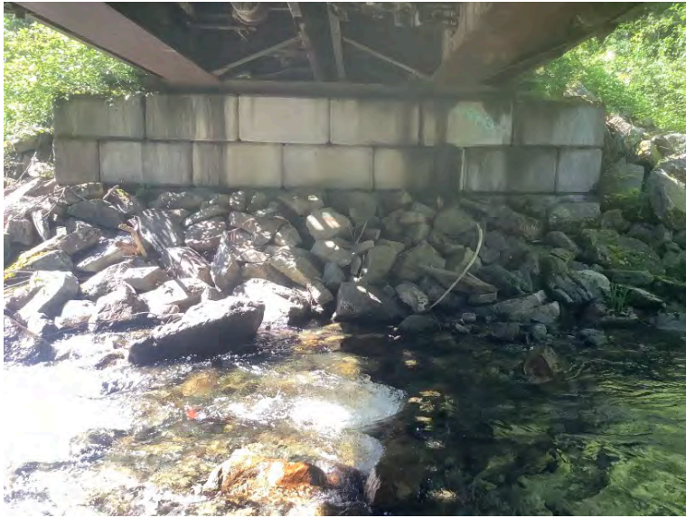
Right Bank Abutment when facing downstream
