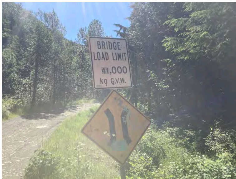
Load Rating Sign
